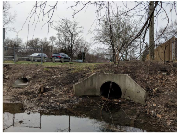
Figure 6: Ingersol Ck, north side 48 inch outlet
