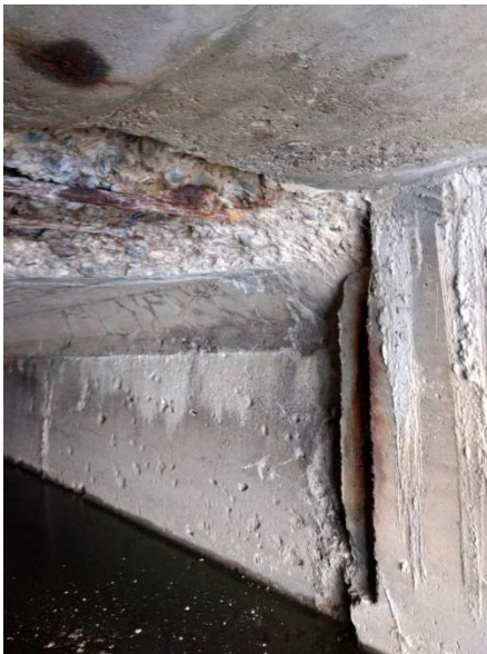
Figure 1: Bishop Ck Culvert south curb line
