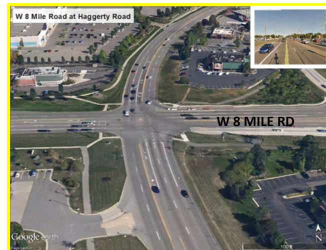
Figure 31. Haggerty Road at 8 Mile Road
