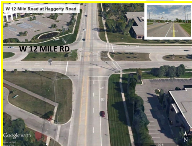
Figure 32. Haggerty Road at 12 Mile Road
