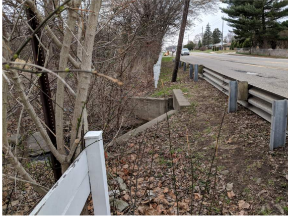
Figure 3: Bishop Ck Culvert, south side looking west
