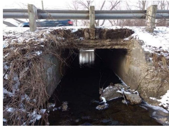
Figure 10: Ingersol Ck Culvert, south side
