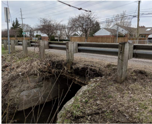
Figure 9: Ingersol Ck Culvert, south side
