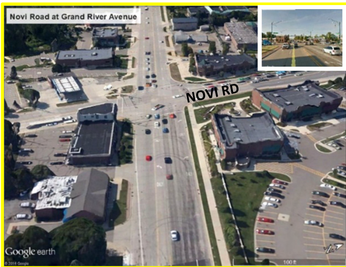
Figure 28. Novi Road at Grand River Avenue
