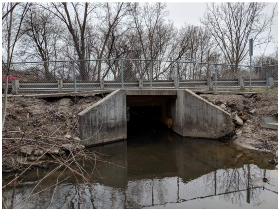
Figure 7: Ingersol Ck Culvert, north side
