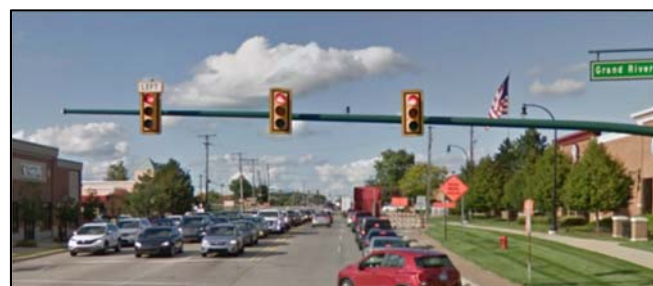
Novi Road and Grand River Avenue intersection with retroreflective backplates already installed on traffic signals.
