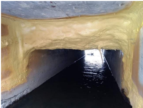
Figure 5: Ingersol Ck Culvert, at north end
